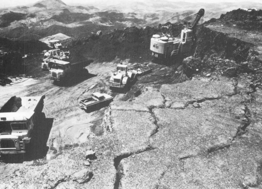
Construction site, Aguas Claras mine near Belo Horizonte, Minas Gerais Courtesy WORLD BANK PHOTO/ Tomas Sennett
