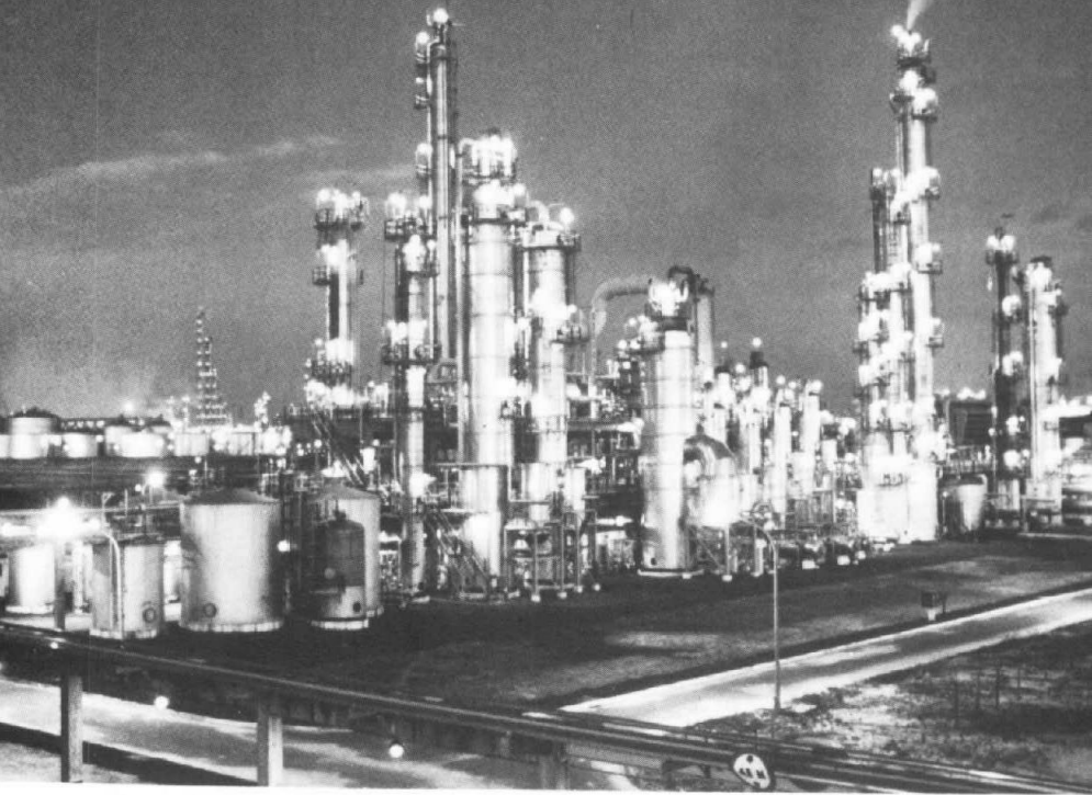
Petrochemical plant, Camacari Courtesy WORLD BANK PHOTO/James Pickerell
