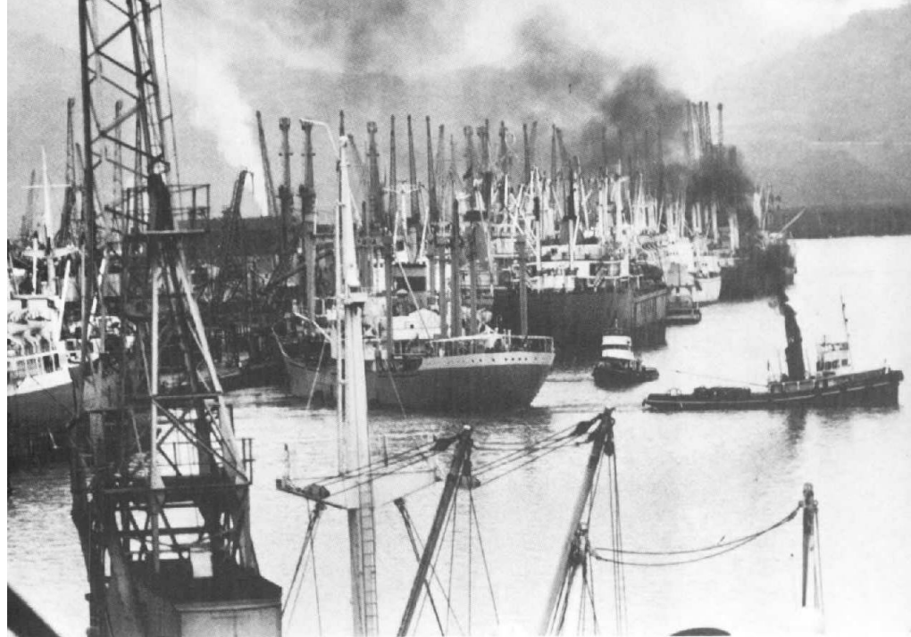
Port of Santos Courtesy WORLD BANK PHOTO/Tomas Sennett
